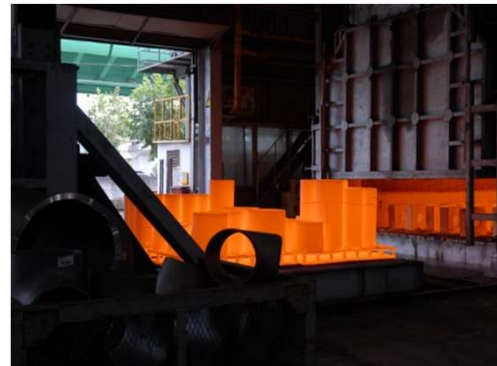
Solution Heat Treatment Furnace
